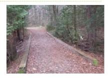
Edge protection **does not** need to be provided if the trail **is not** adjacent to water or a drop-off.
